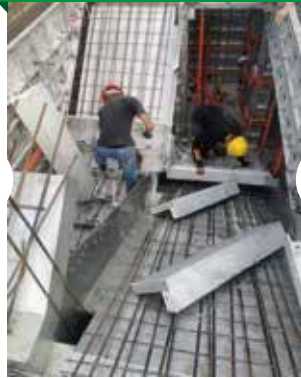
Staircase Panels setup
