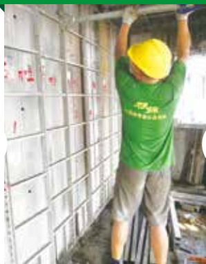
Wall Panels dismantlement
