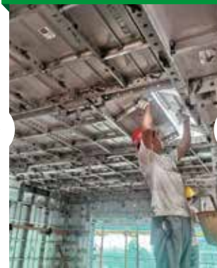
Slab Panels setup
