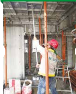
Slab Panels dismantlement
