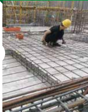
Installation of M&E, rebar
