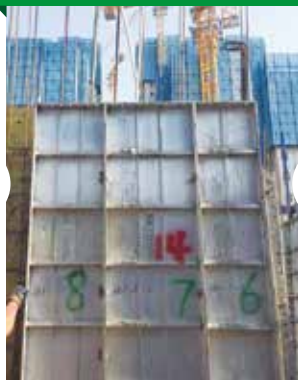
Wall Panels setup
