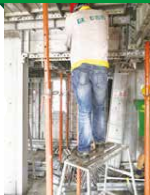
Beam Panels dismantlement
