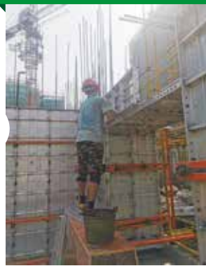
Beam Panels setup
