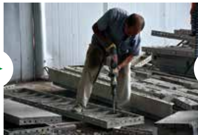
Step 2: Concrete Cleaning
